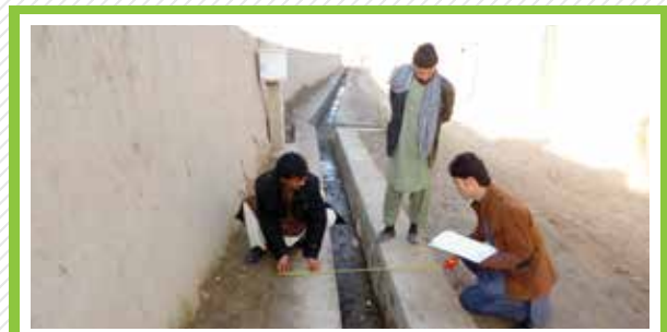
Canal Construction, Khuja Sabz Posh, Faryab
